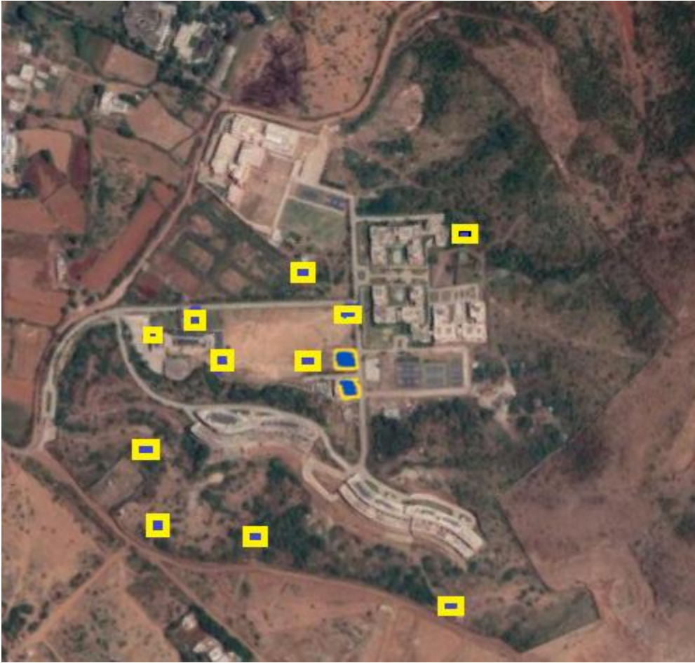
Figure 1: Location of rainwater harvesting pits
